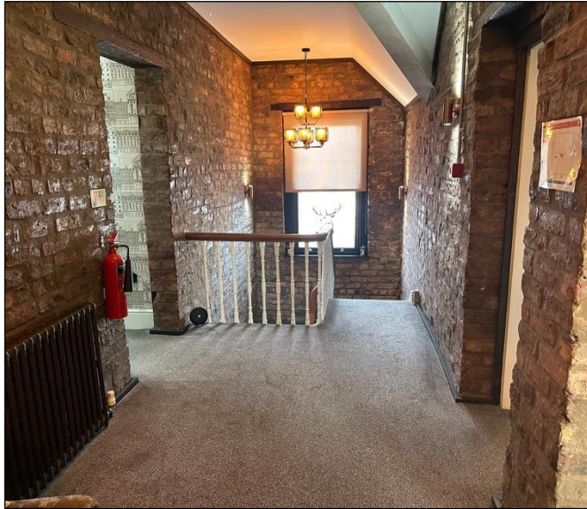
Hotel Entrance, Stairwell & Reception Area
